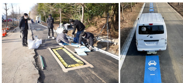
(a) During coil installation (b) After burial
